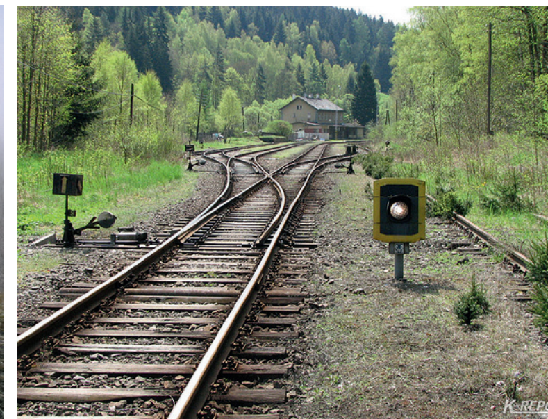
Left picture: Points with a resetting operating mechanism (Photo: Tomáš Lajbl, http://vlaky.bestsite.cz )
