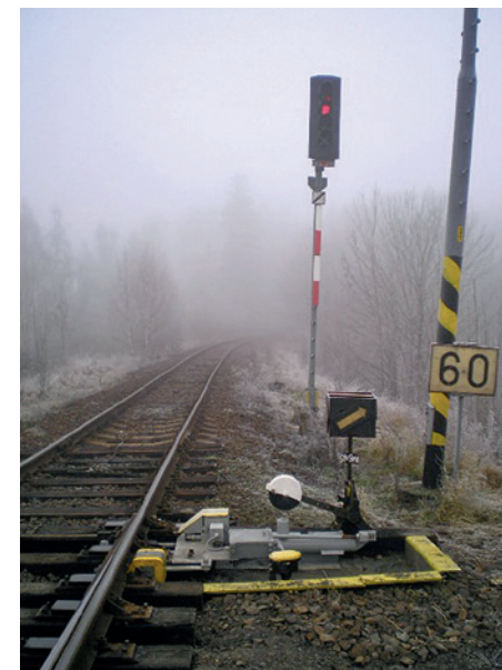
Left picture: Points with a resetting operating mechanism (Photo: Tomáš Lajbl, http://vlaky.bestsite.cz )
