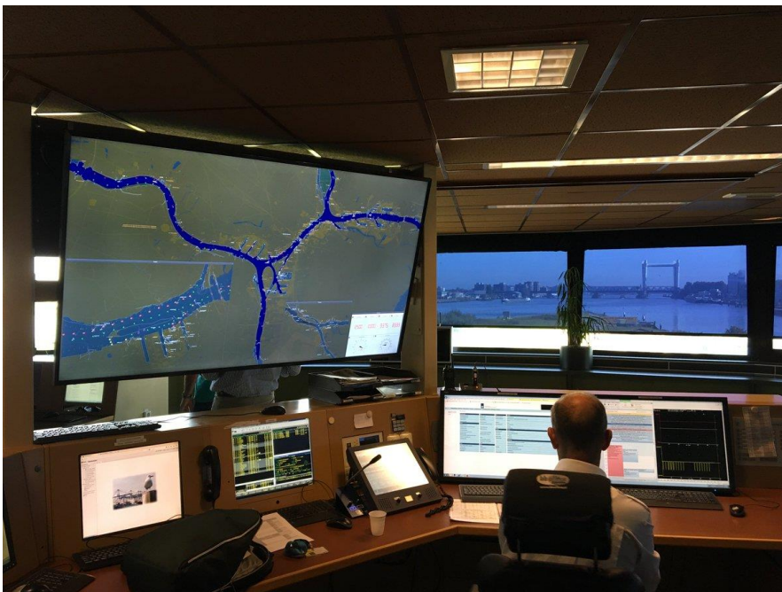
Figure 18: Digitally supported traffic management (source: Rijkswaterstaat)
