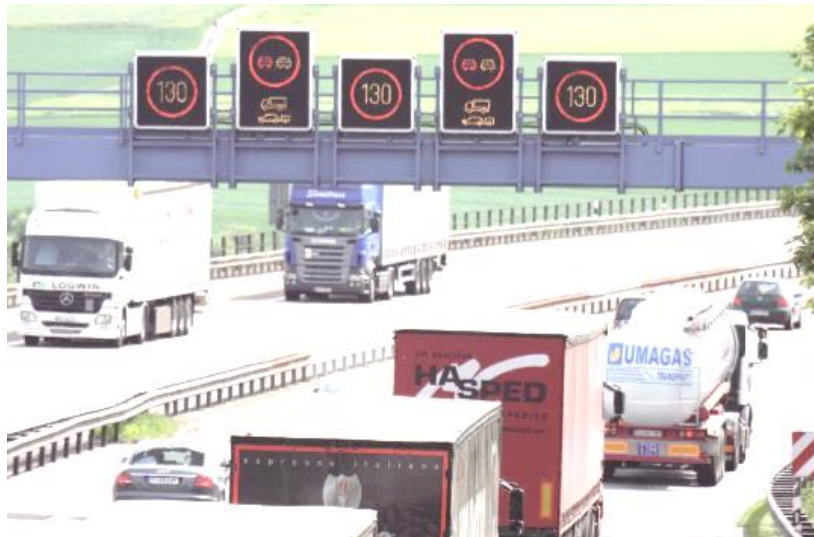
Figure 21: Variable message signs; DATEX II provides the tools for harmonised modelling and exchange of the information displayed
