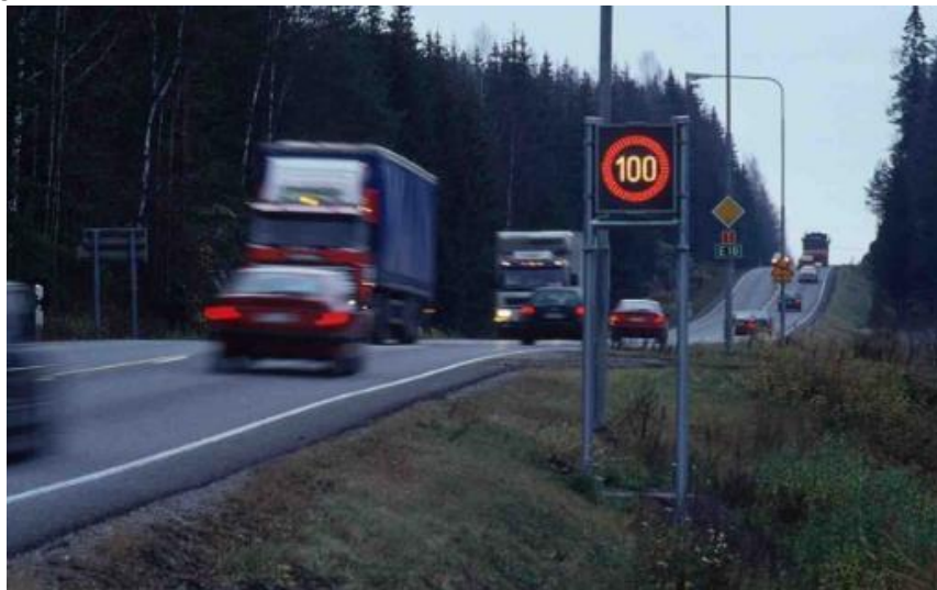
Figure 11.3: Weather controlled Variable Speed limits (source: FTIA)
