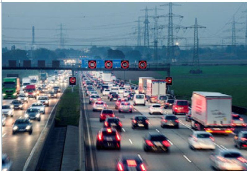
Line control with integrated HSR in operation (A3 Limburg)
