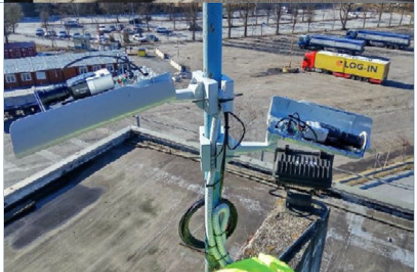
Video surveillance system of ITP Sadobre installed at the roof of a building
