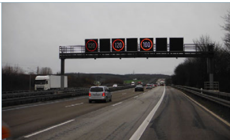
Line control with integrated HSR in operation (A3 Limburg)
