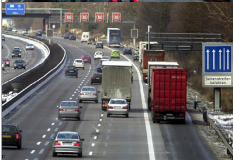
Line control with integrated HSR in operation
