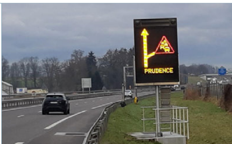
Dynamic safety signage on sensitive spots to faster alert the motorists in case of any queue occurring ahead
